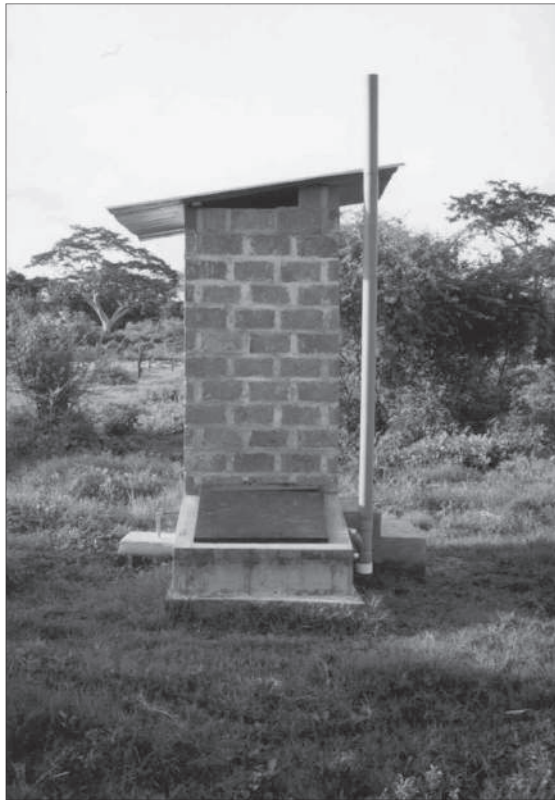
Photograph 5.1. Solar urine-diverting latrine in El Salvador
