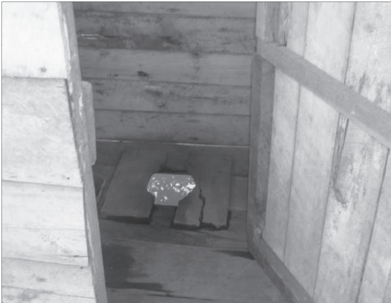
Photograph 6.1. Floating latrine in Indonesia
